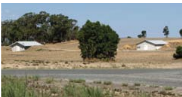
Magazines showing separation and mounds
